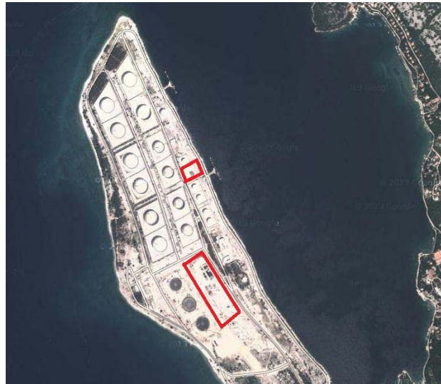
Position neuer Tanks , Kap Tenka
