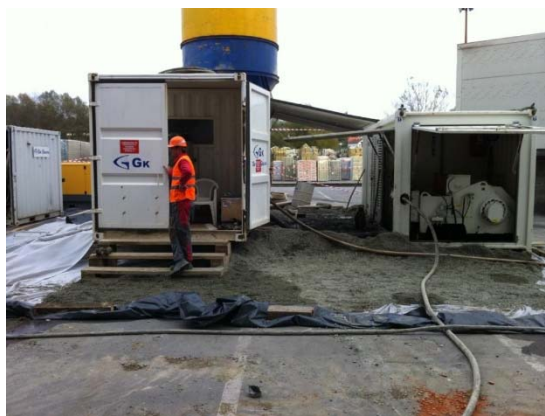
Jet Grouting Anlage
