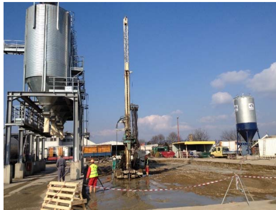
Baustelle Jet Grouting
